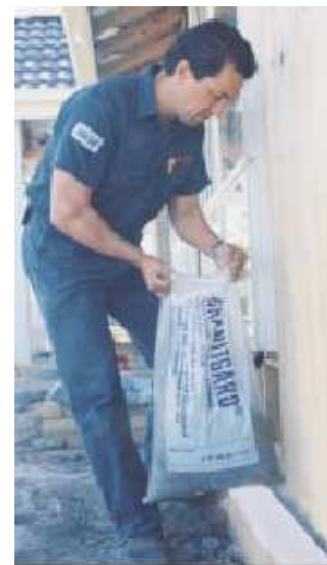
The simple process of installing Granitgard stone.
