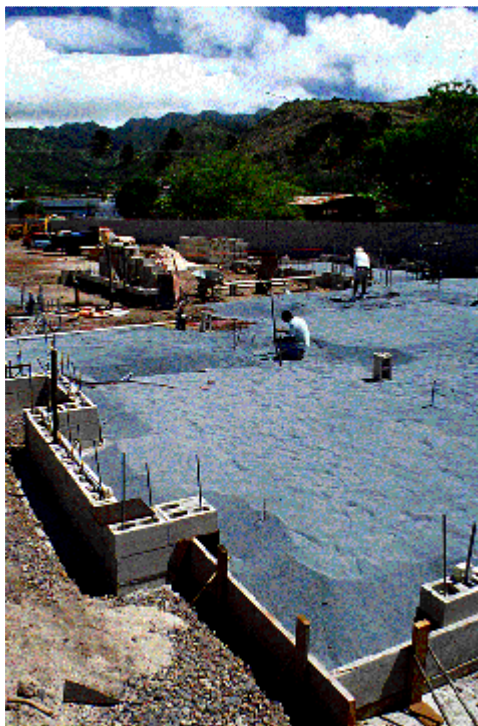
Laying down the BTB. (Photo courtesy of Ameron HC&D.)
